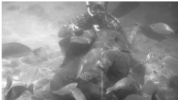
Fig.5. Installation of concrete matrix covered by \text{SrAl}_2\text{O}_4:\text{Eu}^{2+} , \text{Dy}^{3+}
