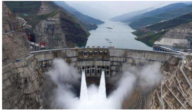
Figure 5. Baihetan Hydropower Station, China[11]
