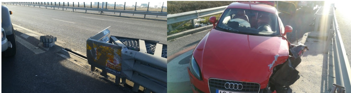
Figure 7. Degraded impact attenuator.
