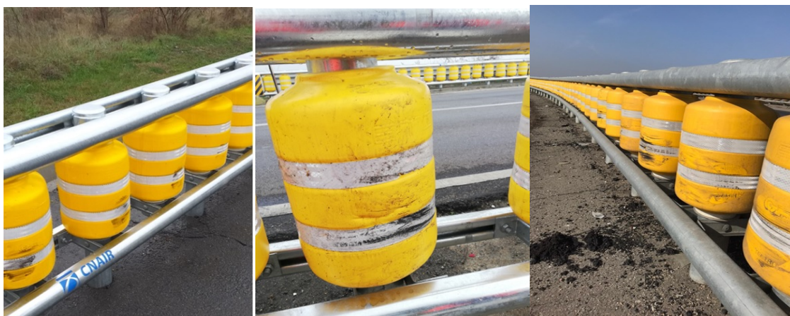
Figure 6. Roller guardrails that took over the road event.
