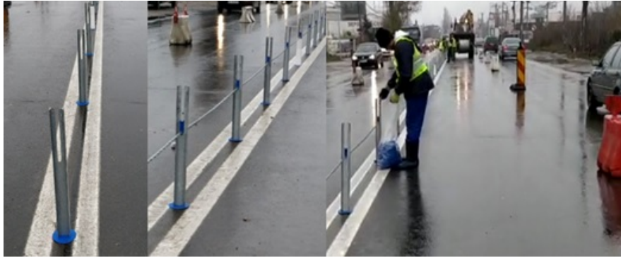
Figure 9. Sector on DN 2 with the cable parapet pilot project.
