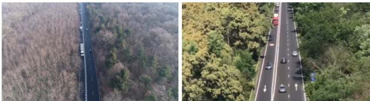
Figure 8. Sector on DN 2 in 2+1 traffic system.
